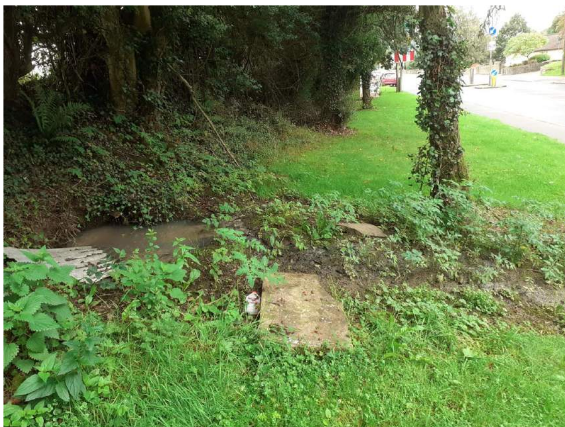
Photograph 6: Overflowing manhole with tomato plants growing in seepage area. (TN7)
